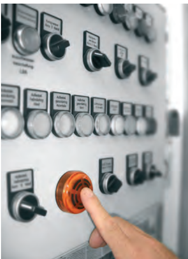
The audible signal can be turned off in seconds by lightly pressing the front of the product
